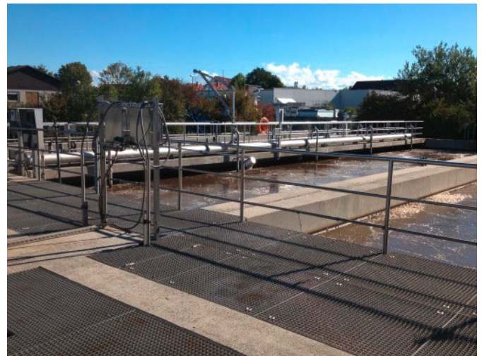
"Two lane" layout of the wastewater plant
